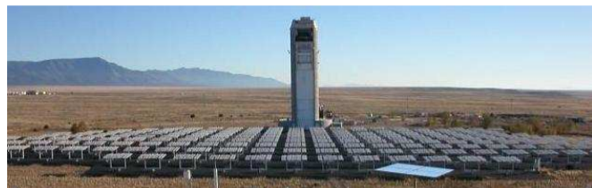
Figure 1: Photograph of the NSTTF in Albuquerque, New Mexico, showing the heliostat mirrors and the central receiver tower. STACEE uses the heliostats and tower as part of a showerfront-sampling atmospheric Cherenkov telescope.
